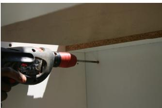
When the cupboard is in the correct position, drill a 6 mm hole through the cupboard and into the wall with a masonry drill. Hammer in a 6x50 mm through-hole-wallplug into the hole, securing the cupboard to the wall. Do this in each top corner of the cupboard. Repeat this as you continue fitting the cupboards in position.
