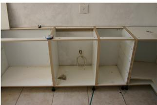
The centre cupboard will house an under-counter oven. Here the backing board of the cupboard was removed to allow the cable into the cupboard as well as to give more depth to the cupboard when fitting the oven. Alternatively, cut a hole in the backing board with a hole saw, to allow the cable through.
