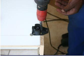
Note that the base plate is fitted with the lip protruding beyond the side. The adjacent cupboard will share the leg with this one. CAUTION!: If you fit the base inside the vertical upright of the cupboard, there will be no adequate support for the cupboard and downward pressure on the cupboard will cause the vertical side to move down and will break out the shelf!
