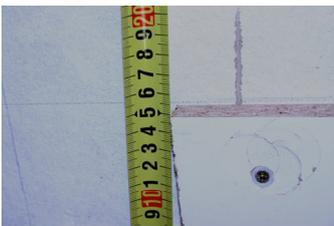
Start by measuring 150 mm up from the floor and marking that on the wall. At this level the cleat carrying the cupboards must be fitted. Use a spirit level to ensure that the cleat is fitted level. When the floor is out of level, start by fitting the cleat at 150 mm at the lowest point of the floor and then working your cleat level to the other end of the wall where the floor units will be fitted.
