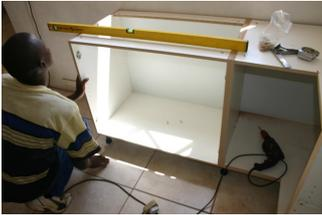
Using a spirit level, check if the cupboard is level, adjust the leg by turning the leg in or out as required to set the cupboard level. Here you can see the first cupboard that was fitted is a corner unit.
