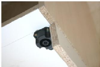
This is a view from the bottom of the cupboard showing how the side kickplate act as a support for the vertical upright of the cupboard. Make sure that the leg is fitted to the base before the cupboard is placed in position.
