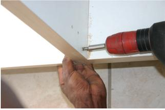
Screw the two fitted cupboards together with a 6x30 mm chipboard screw. Make sure that the cupboards are flush at the front, the top and the bottom. Do this in all four inside corners of the cupboard, two at the front and two at the back.
