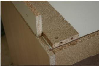
A scrap offcut piece of chipboard is screwed onto the base of the cupboard, set back 20 mm to allow the side kickplate to be fitted against it. This view is from the rear of the cupboard.
