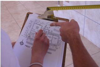
If you have not, in the planning stage, marked out the cupboard positions on the walls, it is advisable to do this before starting to install the cupboards. From the kitchen plan layout take the cupboard dimensions and mark this on the wall where the cupboards will be fitted. This is a check to see if the units will fit as planned. If there are any problems, take care of them now. If everything will fit as planned, you are ready to start with the installation.
