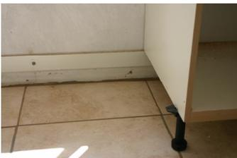
Fit the adjustable leg into the leg base and place the cupboards in position, resting the rear of the cupboard on top of the cleat against the wall. The first cupboard will have two support legs and all intermediate cupboards will only have the one leg sharing with the neighbouring cupboard. The last cupboard in the line will again have two legs. If you have corner cupboards in the design, start with the corner cupboards and work away from them.
