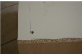
Next start fitting the plastic support legs to the bottom front of the floor units. Unclip all the doors from the cupboards, this makes them easier to handle and to install. Turn all cupboards upside down. Mark 50 mm from the front of the cupboard, this is where the leg base will be fitted. Screw the adjustable leg base plates down with 6x16 chipboard screws.
