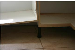
Continue placing the cupboards next to each other, fit the through-hole wallplugs, screw the cupboards together and check with the spirit level and adjust the legs as required until the last cupboard is placed in position. Remember the last one has two legs, with the outside leg fitted as described above, the side kickplate supporting the vertical upright of the cupboard.
